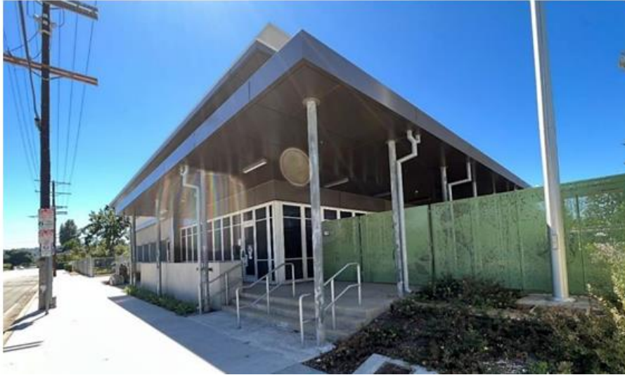
Colfax Charter ES Classroom Addition Project – Main Entrance Area Gate
