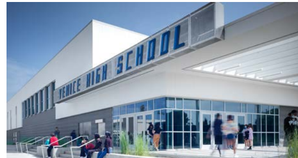
Venice HS Comprehensive Modernization
