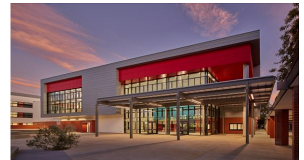
Cleveland HS Comprehensive Modernization
