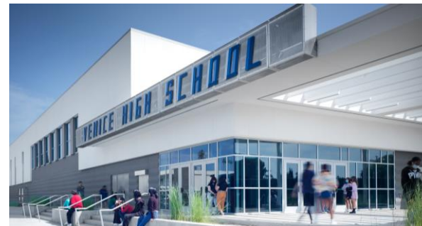
Venice HS Comprehensive Modernization
