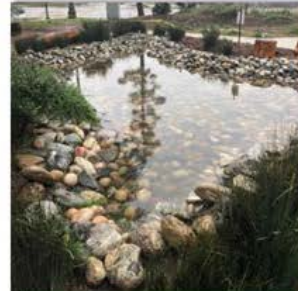
Carthay Environmental Magnet School's bioswale captures rainwater and prevents flooding in an area that was previously grass.
