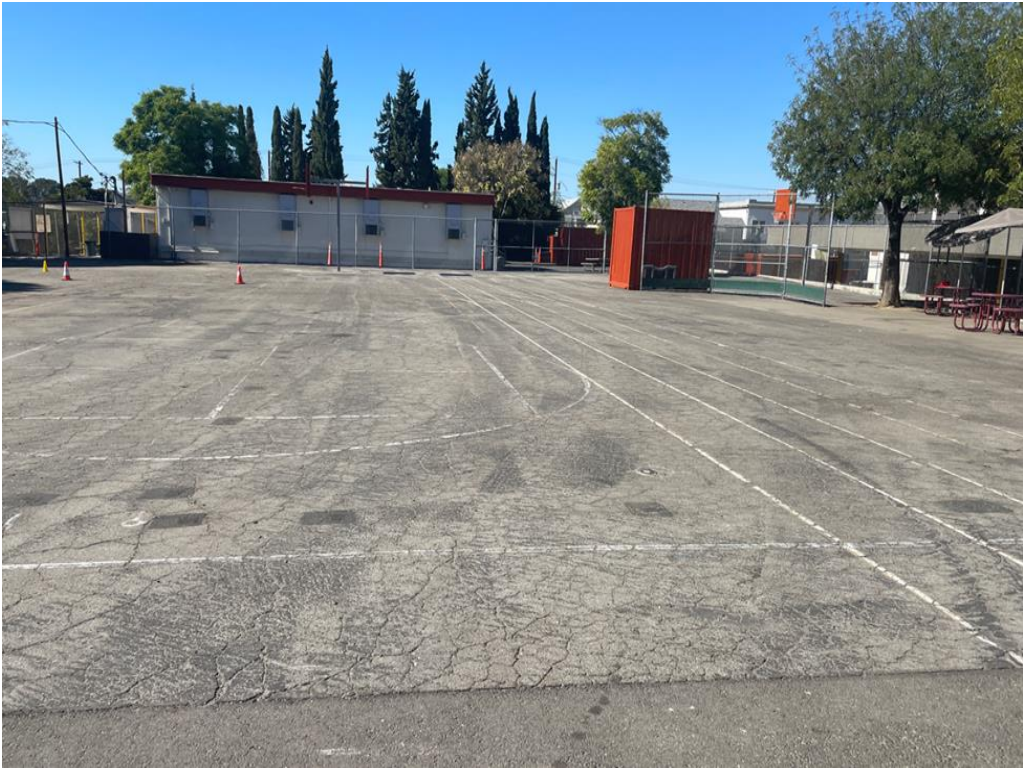
South playground looking west
