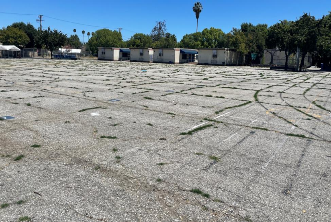
Playground looking southwest
