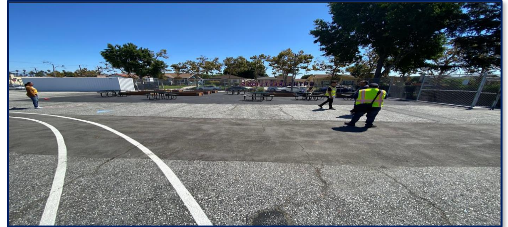
Location for Shade Structure
