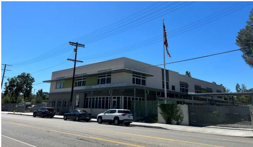
Main Classroom Building – Entrance View
