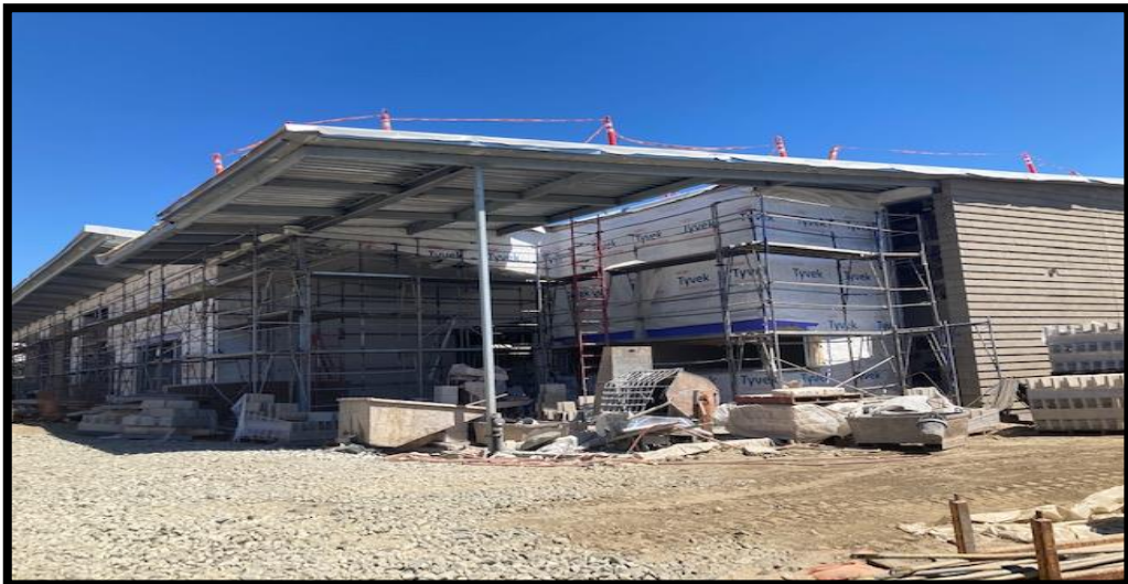
In Construction: New Administration & MPR Building
