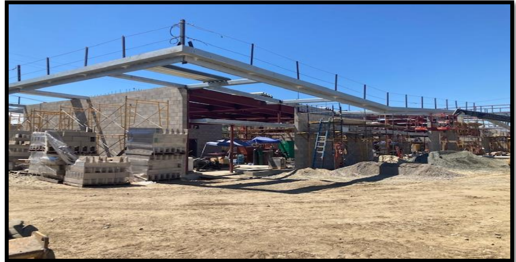
In Construction: New Classroom Building
