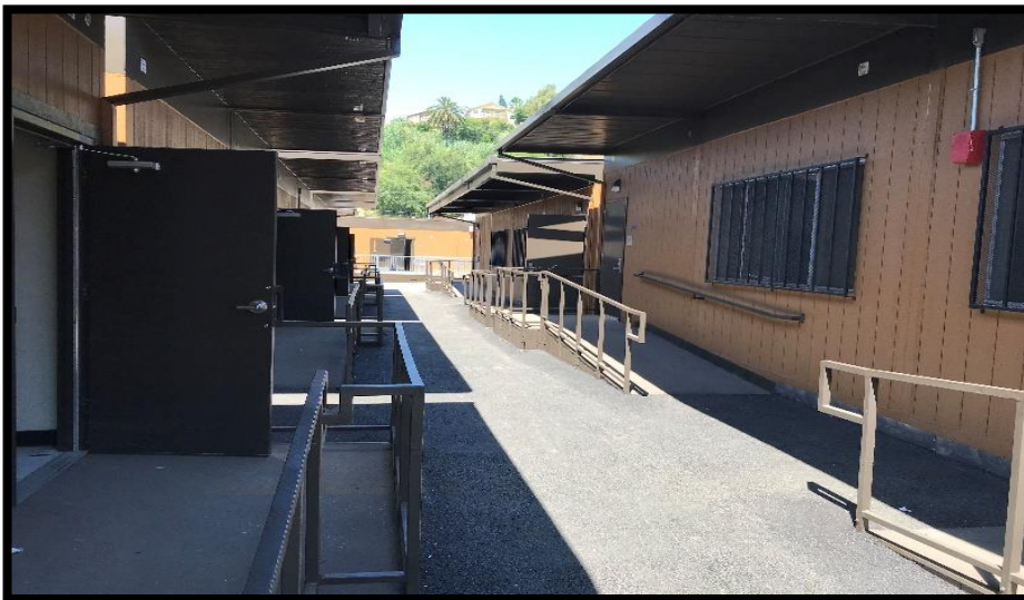
In Construction: Interim Housing Village
