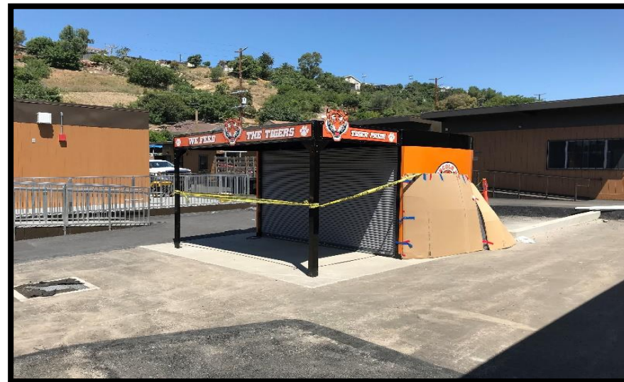
In Construction: Student Store Kiosk
