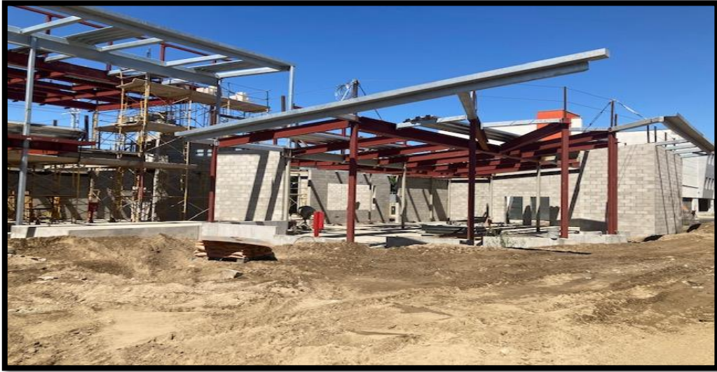
In Construction: New Classroom & Library
