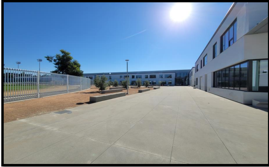
Completed: New Classroom Exterior and Hardscape
