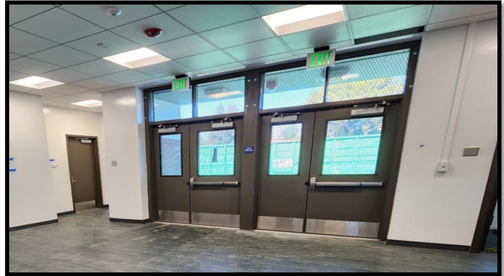
Completed: North Gym Interior Entrance
