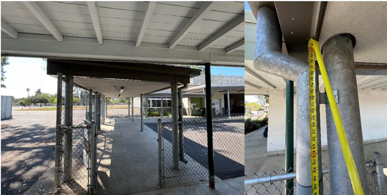
Kindergarten Walkway Canopy – View of Entry and Canopy Height Measurement (OIG Photo – 9/6/2022)
