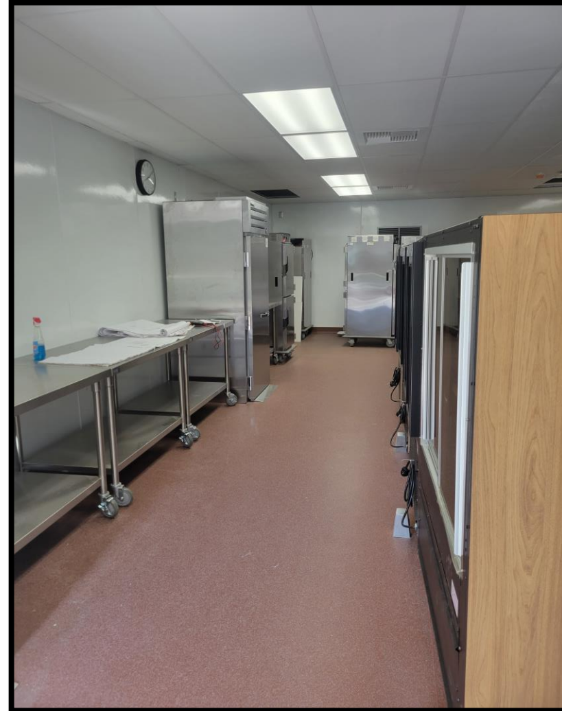
In Construction: Interim Kitchen Scramble
