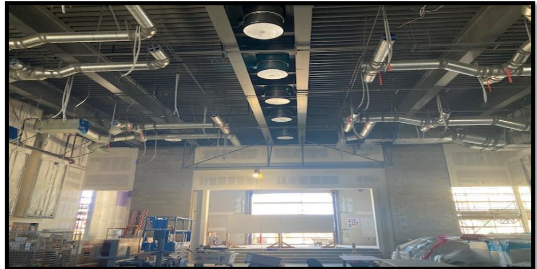
In Construction: New MPR
