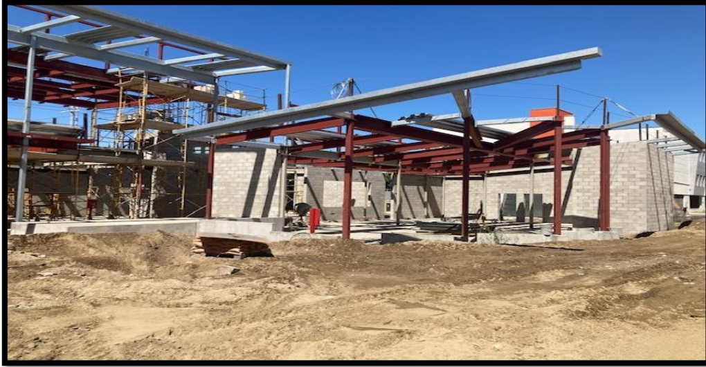
In Construction: New Classroom & Library
