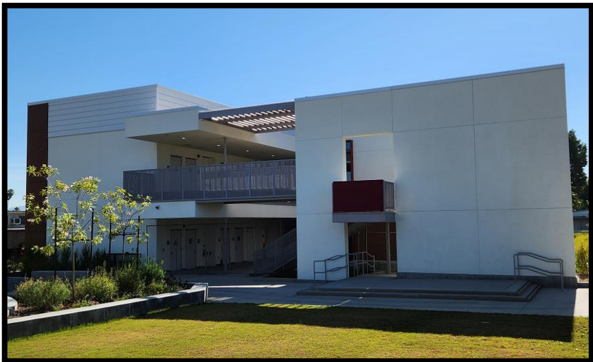
Completed: New Science Building West
