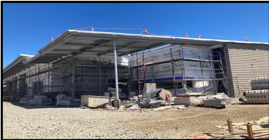
In Construction: New Administration & MPR Building
