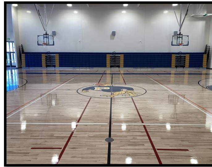
Completed: Basketball Court
