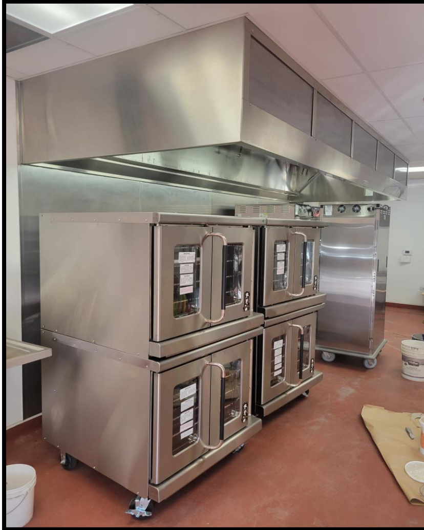
In Construction: Interim Kitchen
