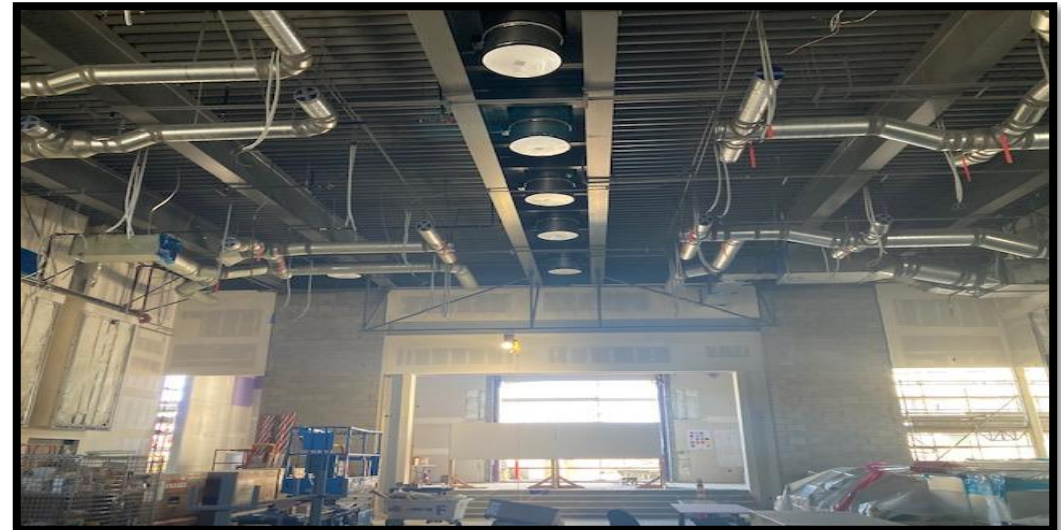
In Construction: New MPR
