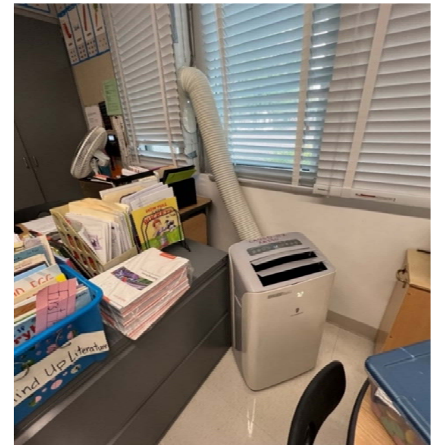
Colfax Charter ES Classroom 127 Portable Air Conditioner Unit Installation (OIG Photo – 10/22/2022)
