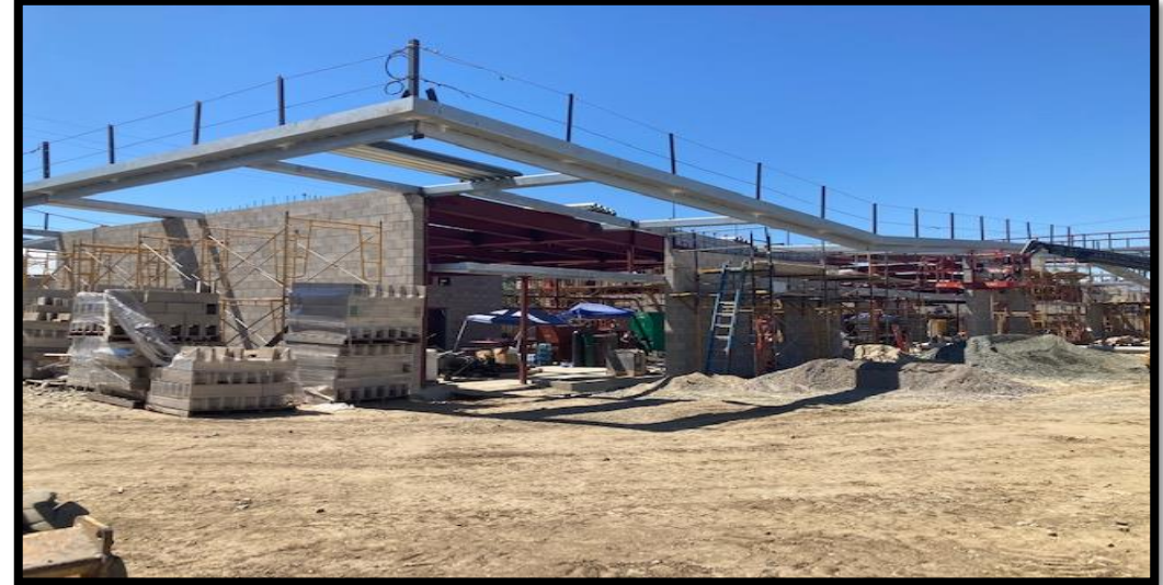
In Construction: New Classroom Building
