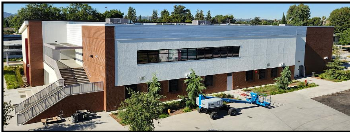
Completed: New Science Building West
