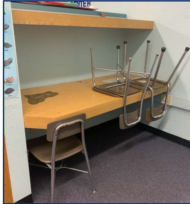
Built-in Desk to Remove and Replace with Shelving
