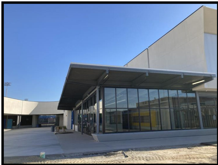
Completed: Gym Exterior
