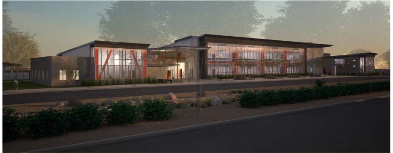
View Looking From Drop-Off Round-About To Middle School Entry Breezeway
