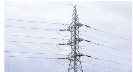
This is a power grid.
