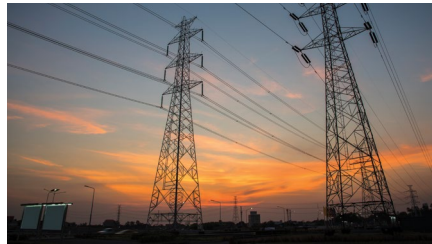
This is a power grid.
