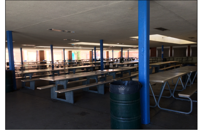
Photo 9. View of outdoor dining area adjacent to Building 23 (Cafeteria).
