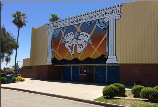
Photo 4. View of Building 1 (Auditorium) entrance looking south.
