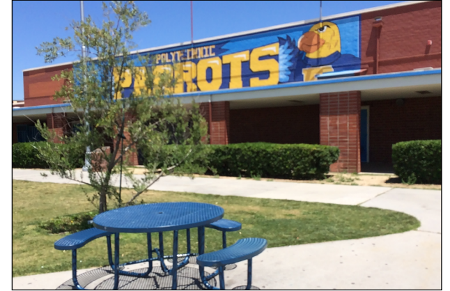
Photo 3. View of Building 23 (Cafeteria) looking north from the polygon.
