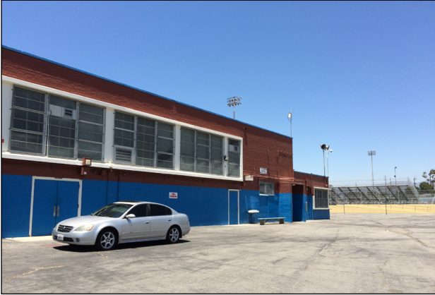
Photo 7. View of Building 45 (Girls' Gymnasium) and bleachers looking northwest.
