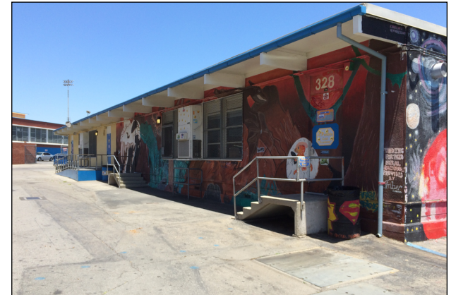
Photo 12. View of Building 32 (portable classrooms) looking north from Building 24 (Utility Building).
