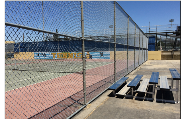
Photo 6. View of tennis courts looking north from Building 45 (Girl's Gymnasium).
