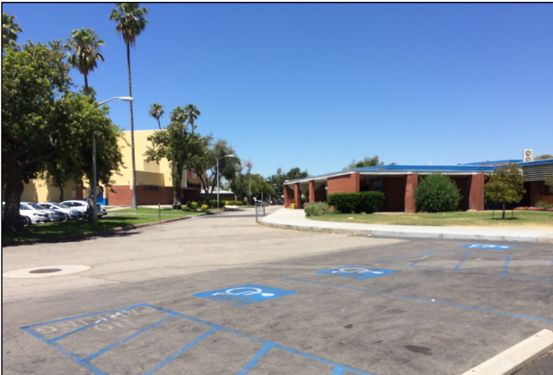
Photo 10. View of Parking P-1.1 looking west toward Buildings 1 (Auditorium) and 10 (Library).
