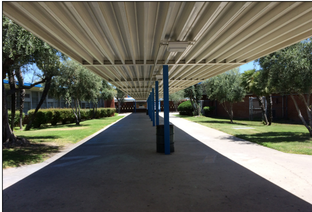
Photo 5. View of covered arcade between buildings.
